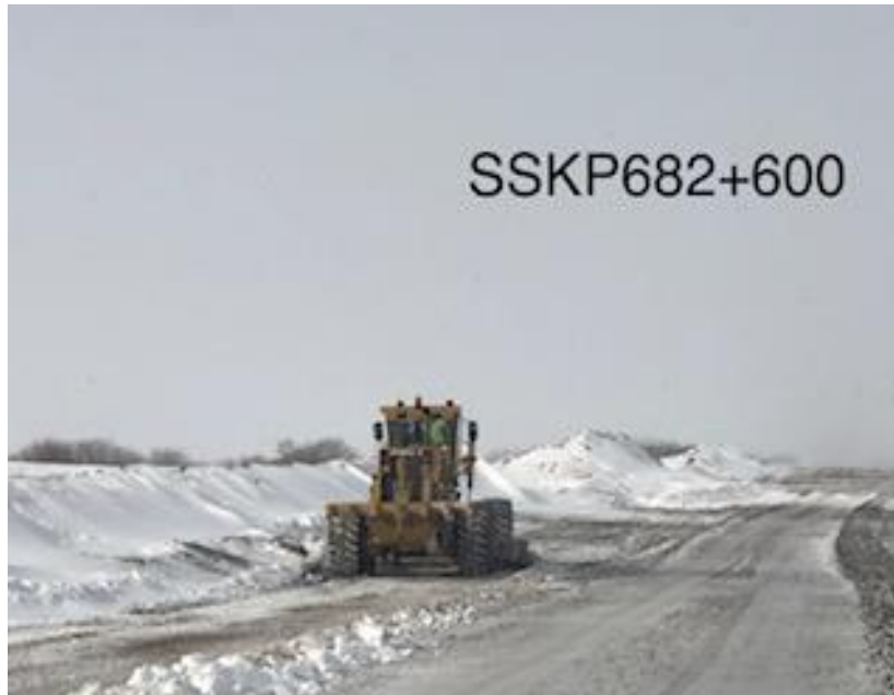
Machine clean up completed on Spread 5 – grading the right of way
