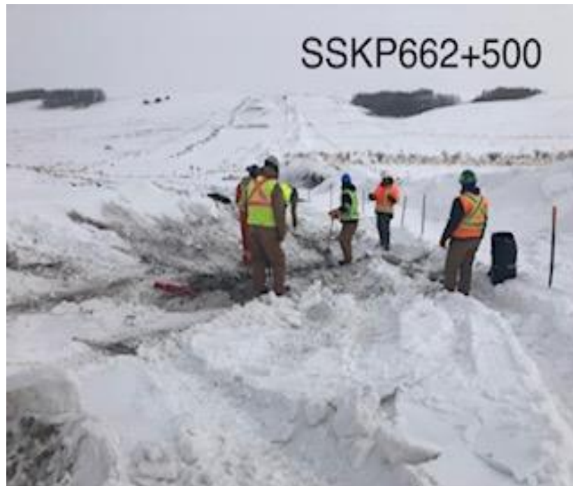
Silt fence installation at water crossing Vipond Creek SK WC72
