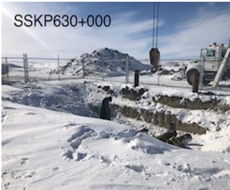
MLBV16 welding extension piles at the valve site
