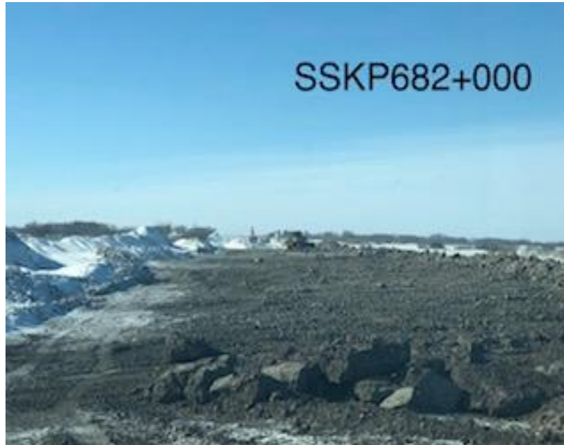
Machine clean up on the right of way
